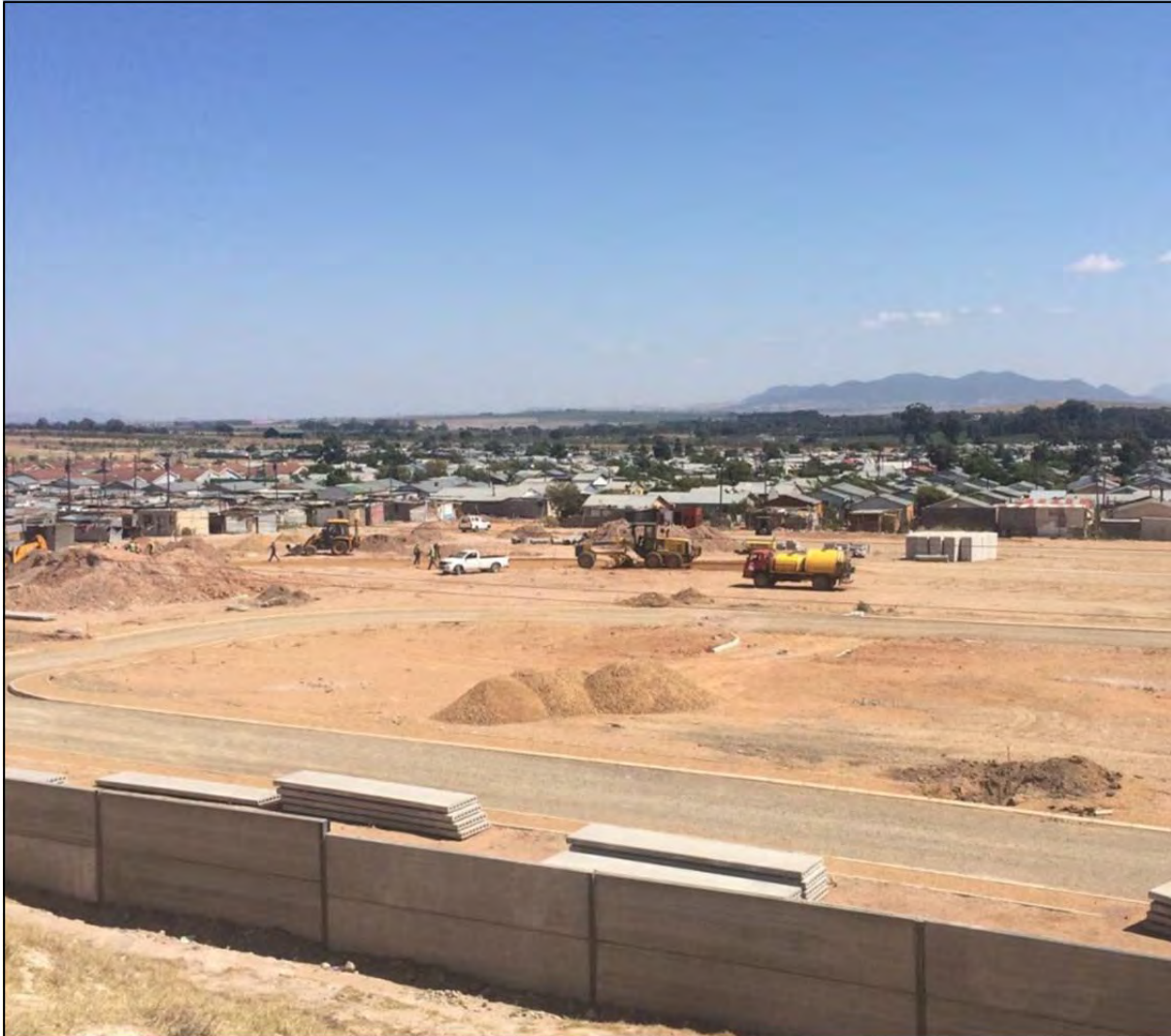
Installation of services in progress.
